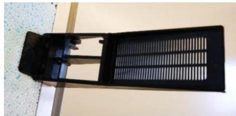
Figure 9 - Soffit bracket fixed on the rail
